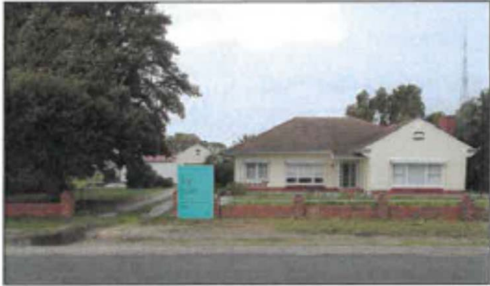
Photo 1 – Allotment 1, East Terrace – existing dwelling and garage buildings
